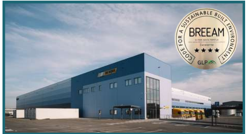
Warehouse in Santa Perpètua de Mogoda
