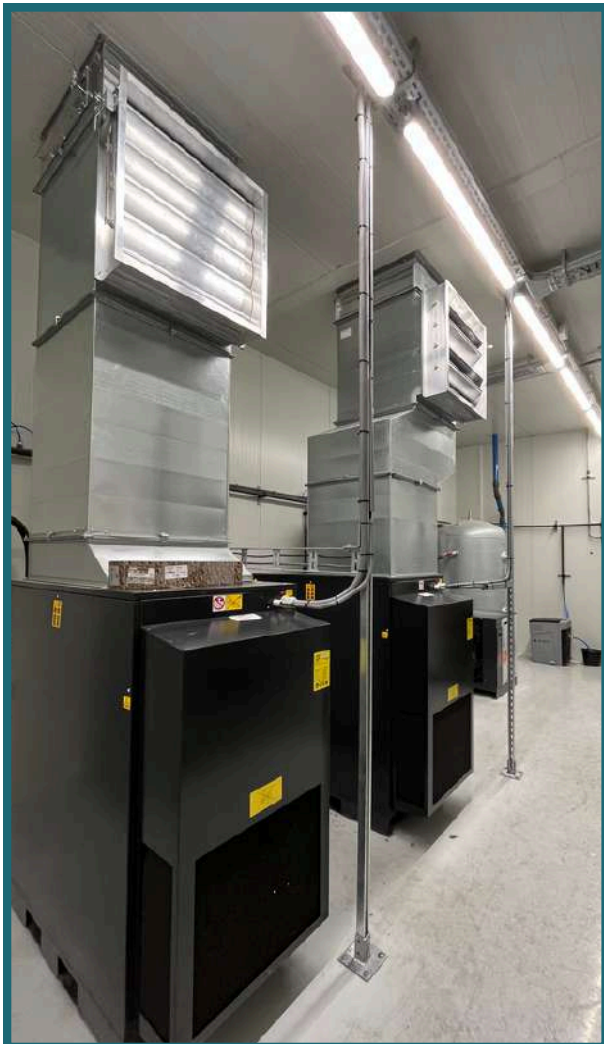
Two frequency-controlled compressors, Warehousing Botlek
